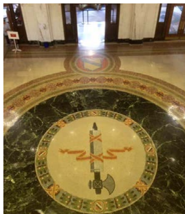
A beautiful inlaid terrazzo marble floor adorned the entrance to the Douglas County Hall of Justice.
